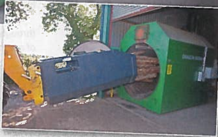
▲ The Dragon biomass boiler heats 30,000 litres of water, which means heat is retained for many hours after the boiler ceases operation.
