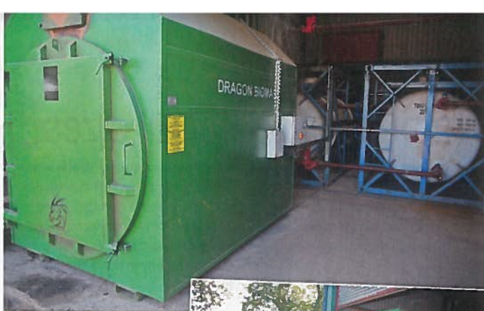
▲ The Dragon biomass boiler heats 30,000 litres of water, which means heat is retained for many hours after the boiler ceases operation.
